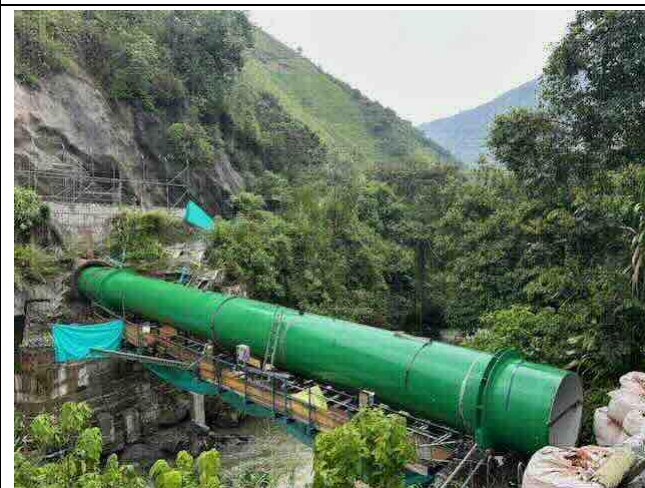
Photo 18: Chorreritas HPP penstock bridging the San Andrés River
