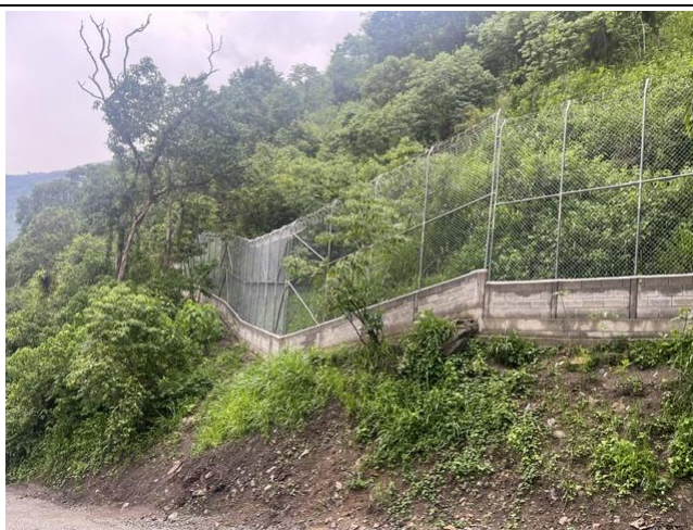
Photo 17: Example for slope protection and fencing, at headworks of Chorreritas HPP
