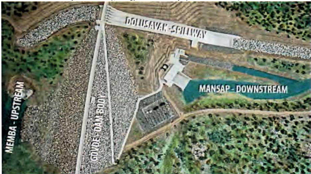
Picture 3 Reconstruction of the dam body, energy tunnels and safety canal
