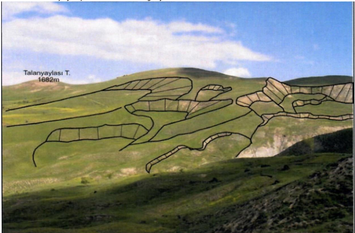
Picture 8 Instability of slopes in the surroundings of Dumlusu
